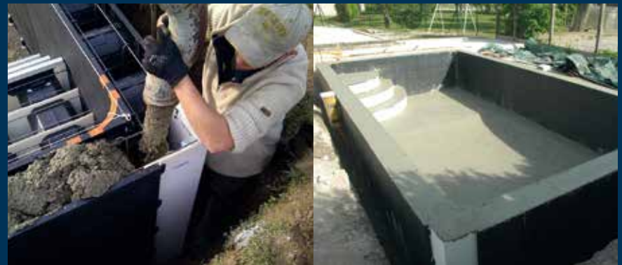
4 - Concrete casting
